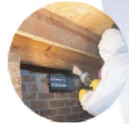
Flat open areas are cleaned quickly with wide nozzles.
