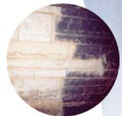
Fire restoration on a residential fireplace.
