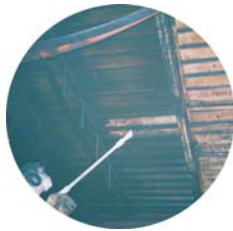
Remove soot and char without increased waste or water damage.
